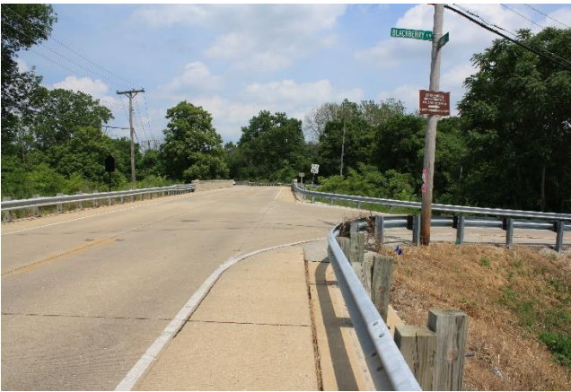
PHASE II Looking East
