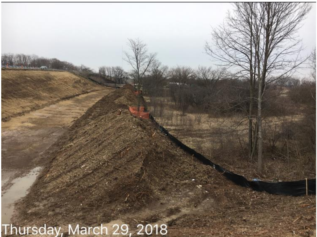
Figure 5: Silt fence in place and in good condition along the west side of I-55, facing east.
