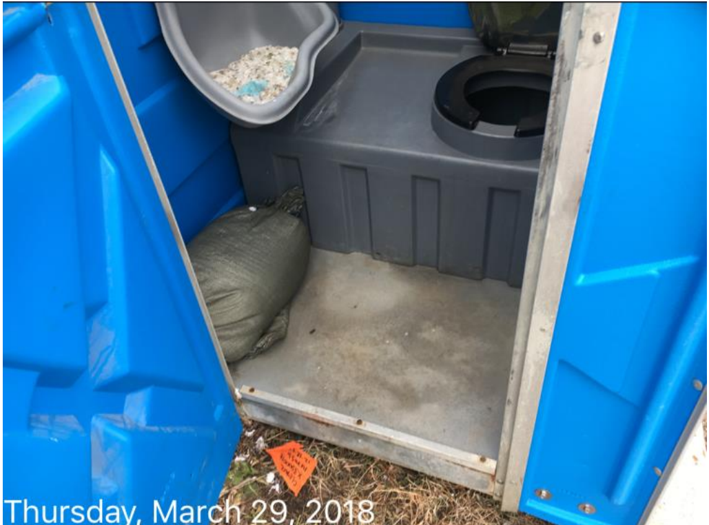
Figure 6: Portable toilet in place and adequately stabilized with a sand bag to prevent it from tipping over.
