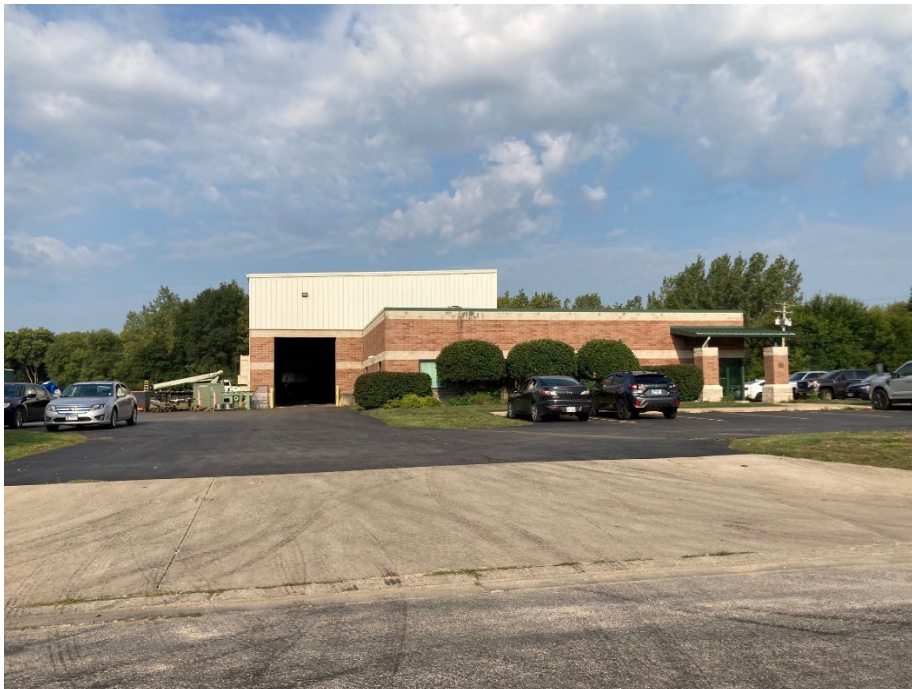
Photo 7: View of existing building from south access drive.
