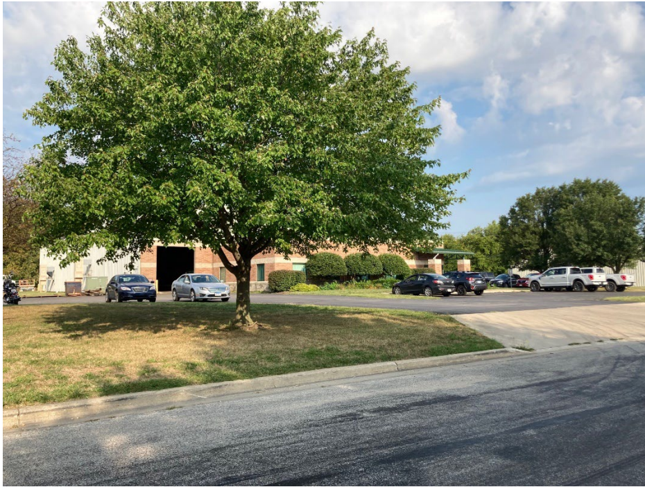
Phot 6: View of existing building and front parking lot from Northern Illinois Drive.
