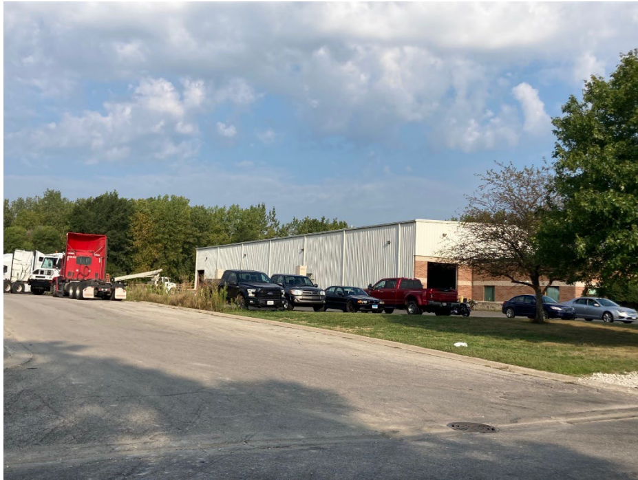
Photo 4: View of south side of existing building.
