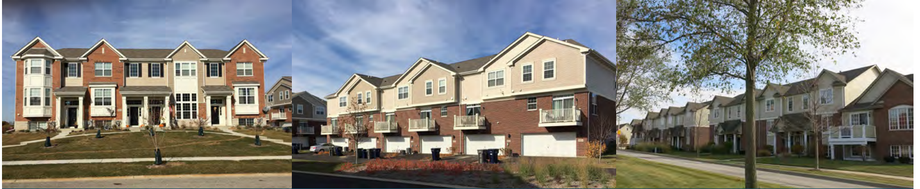
153rd Metra Station TOD, Orland Park (owner occupied)
